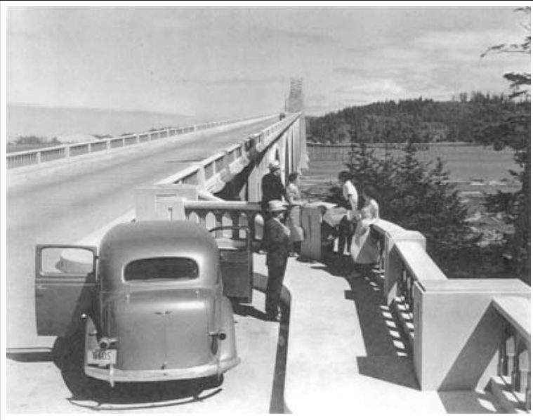
McCullough Bridge at Coos Bay Tourists (Photo Courtesy of Oregon Department of Transportation)
